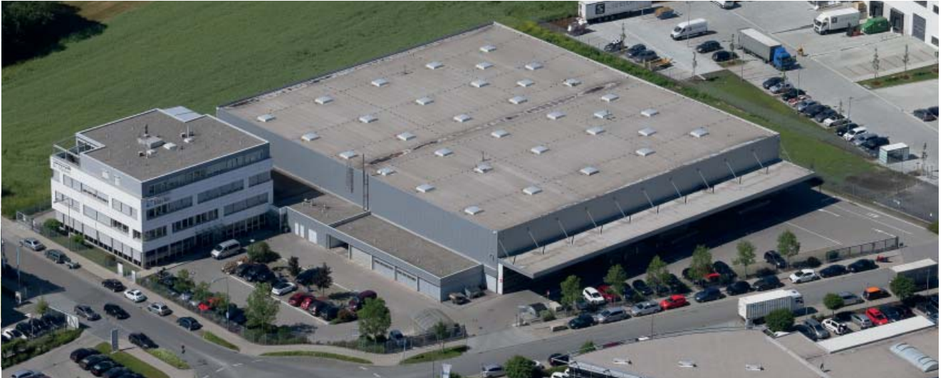
MayTec GmbH plant in Dachau
